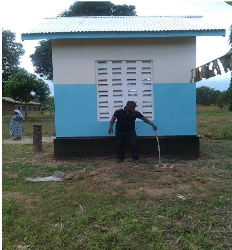
Plate 3: Diesel Generated Pump House in one of the Project in the Study Area
